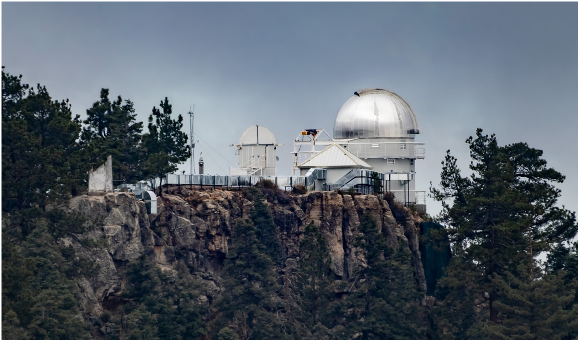
Figure 1. The COLIBRÍ buildings. On the right is the main building with an aluminum dome. The building just to the left of this, with the sloped roof, is the service building. The exhausts for the air-conditioning system extend along the edge of the cliff to the left. The building in the middle, with the clam-shell enclosure, is for the BOOTES-5 telescope. The weather station and seeing monitor are on the column and mast to the left of the BOOTES-5 building.
