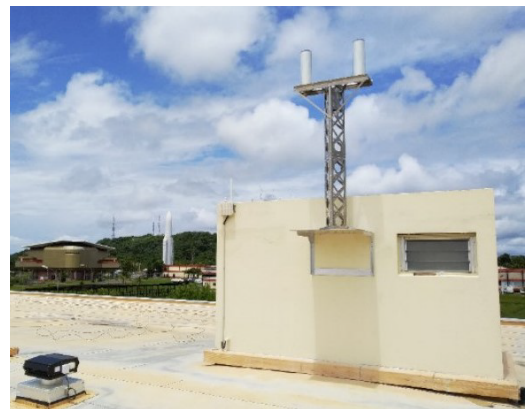
Figure 2. VHF operational ground station in Kourou.
