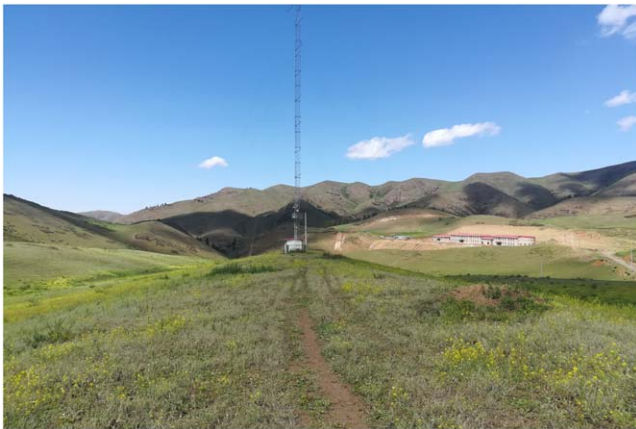
Figure 2. The construction site of Qitai LFRA (The wind tower direction is due north).
