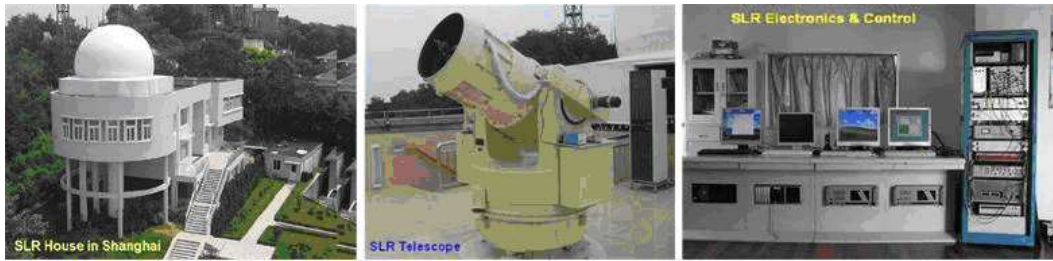
Fig. 2 Shanghai SLR station, telescope and electronics control room.
