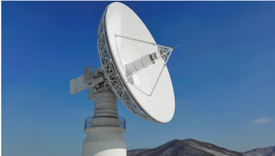
Fig. 3 The 13-m Cassegrain radio telescope at Jilin station.
