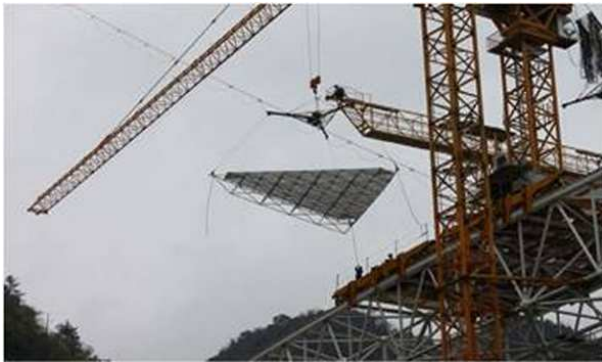
Fig. 7 The first transfer in the air (from crane tower to transfer truck).
