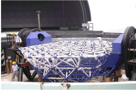
Fig. 16 Ma support structure being installed.
