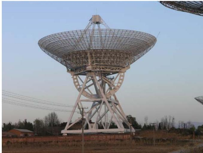
Fig. 12 Fifty-meter parabolic radio telescope at the Miyun Station, NAOC.
